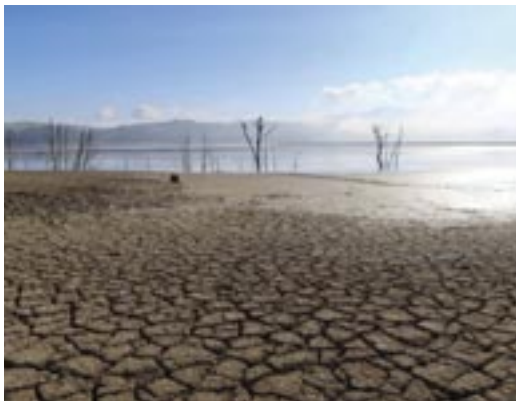
A view of cracked ground near the Sidi El Barrak dam with depleted levels of water, in Nafza, west of the capital Tunis, Tunisia REUTERS/Jihed Abidellaoui
