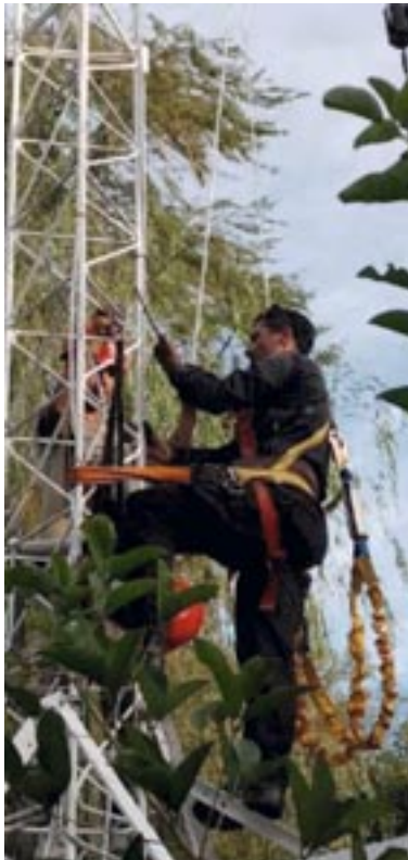
Installation of the new Radio El Libertador antenna
