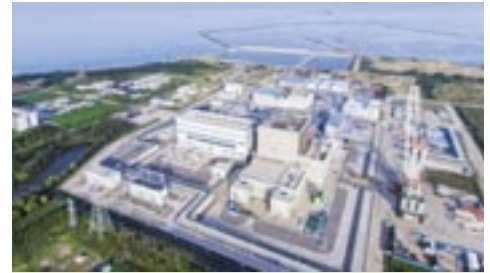
The fourth generation Shidaowan plant in China’s northern Shandong province is designed to use fuel more efficiently. File Photo.
